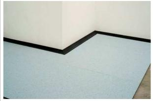
Fit the Colorex Plus tiles tight between the cove and the installed Colorex Plus floor.
