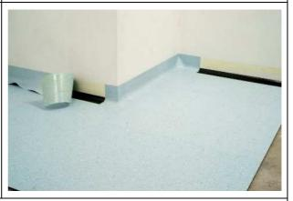
Install the preformed internal and external corner pieces and the cove skirting stripes with contact adhesive.
