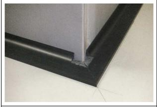
Cut the profile-end to make room for the reinforcement at the back of the Colorex external preformed corner.
